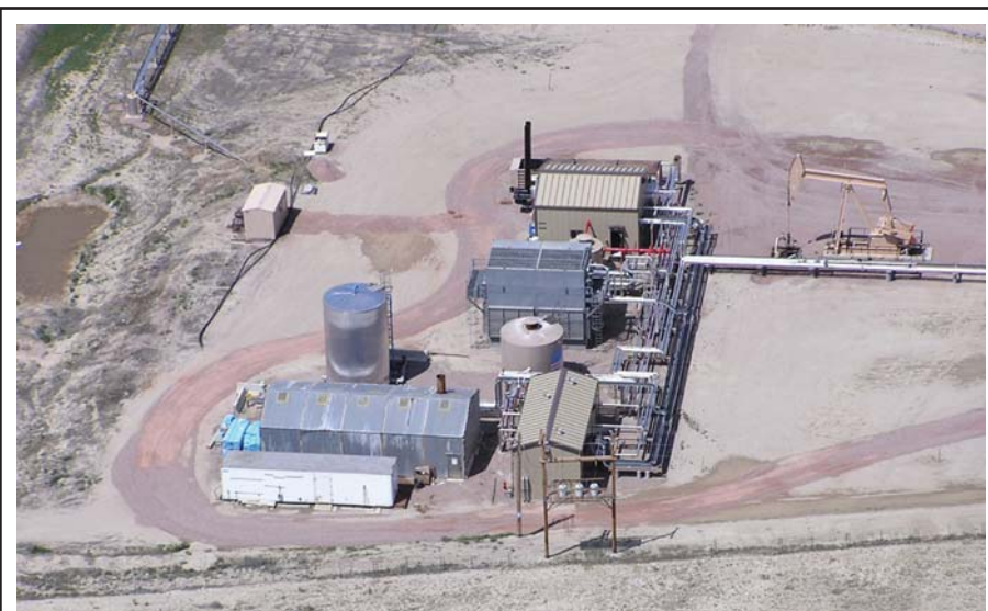
Derek Oil & Gas Corporation and Ivanhoe Energy are jointly developing the LAK Ranch Field, an 8,000-acre property located along Interstate 16 in Weston County, Wy. The project is in the pilot phase of a modified steam-assisted gravity drainage EOR process targeting a high-quality viscous oil in the Newcastle Sand formation.
