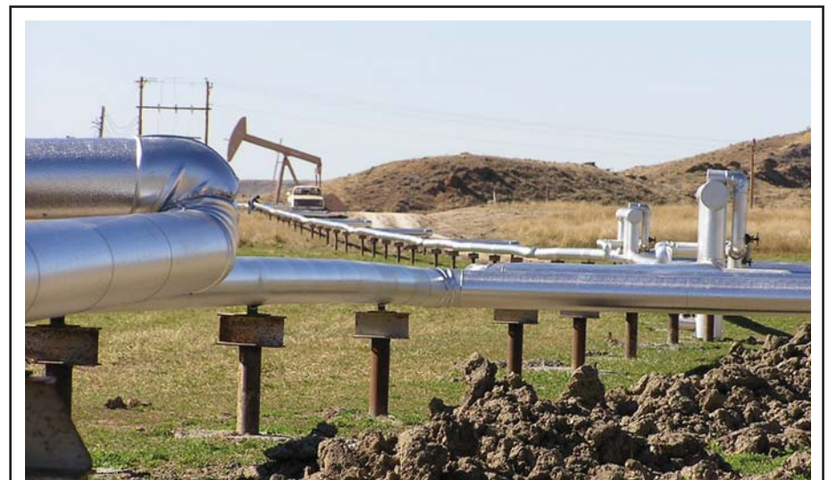
LAK Ranch uses a modified SAGD approach that pairs vertical steam injection wells with horizontal oil production wells, as opposed to a conventional SAGD design using two parallel horizontal wells. Some of the vertical injection wells used in the pilot project are shown here.
