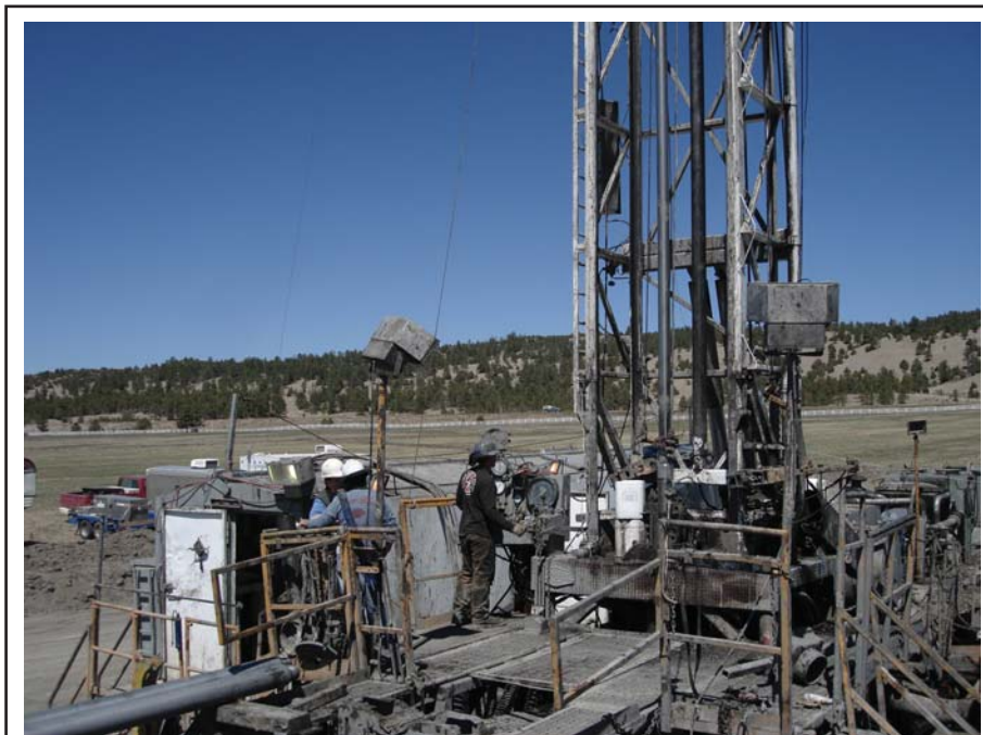
The drilling crew works on one of 12 wells—four injectors and eight producers—Derek Oil & Gas drilled this spring in the initial phase of its LAK Ranch heavy-oil steamflood project.
